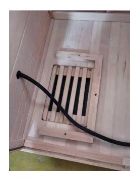
Now that the stove is wired, one person lifts the stove into place and the other gently pull the cable back so there is no excess cable at the bottom.
