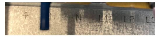
These connection blocks use ring plates. You want the flat side facing down to get a good connection. Tighten the screw in well
